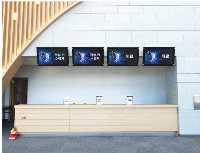
DID(3층 등록데스크, 1,920×1,080 픽셀)
